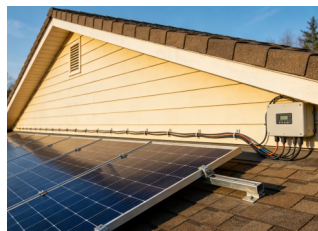
Residential Rooftop PV Systems
