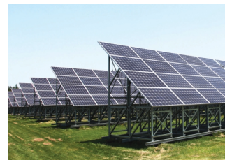
Commercial Rooftop PV Systems
